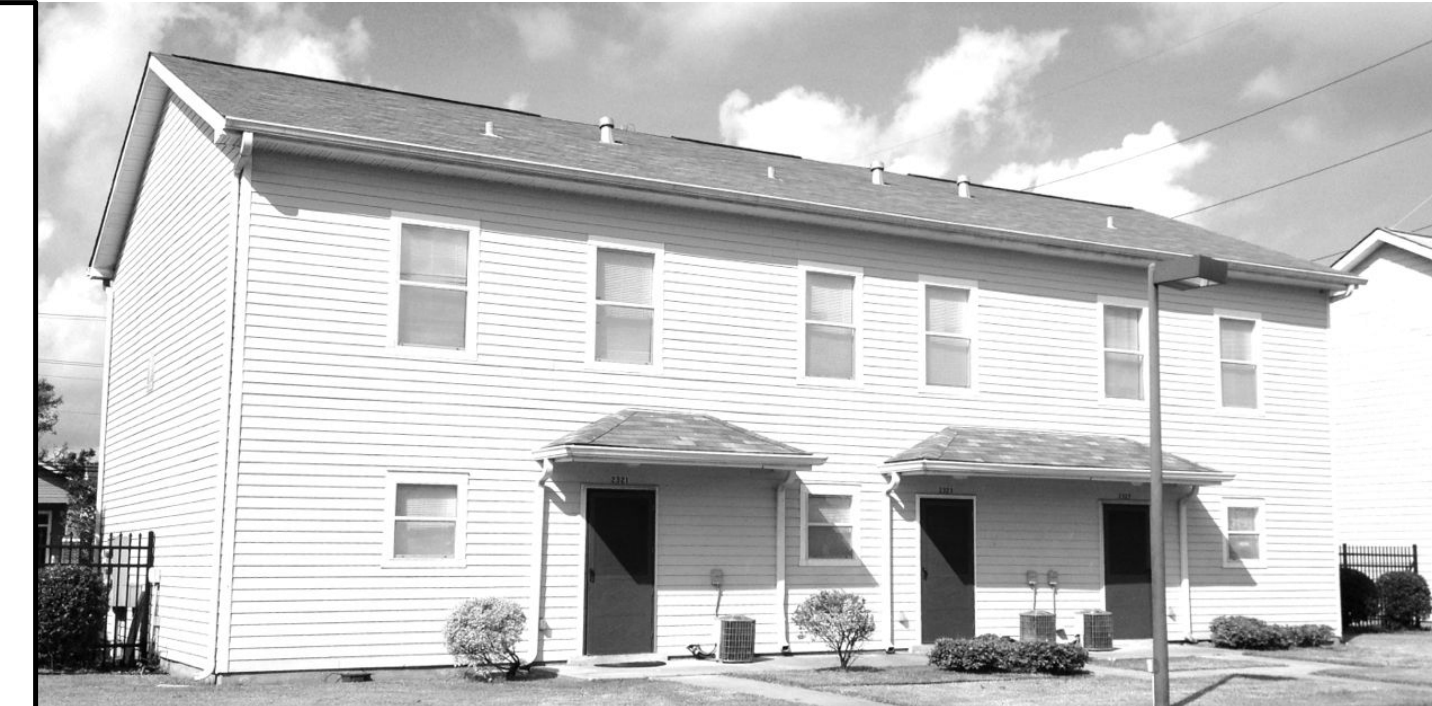
This photo shows the typical rear elevation appearance of Building Types "B", "C", and "D".
