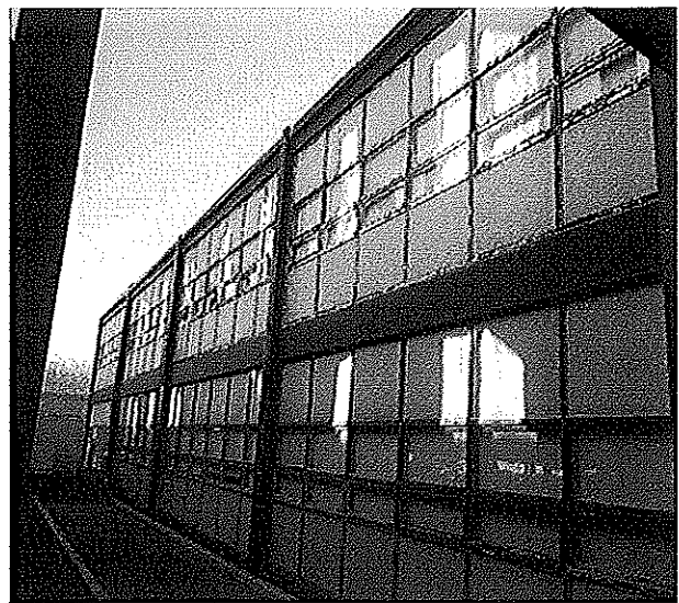
Building B Rear Breeze way
